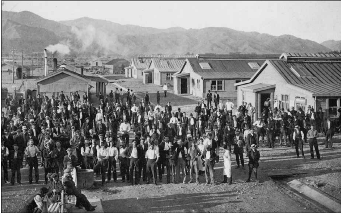
Public Works builders pause beside the cookhouse and dining halls during construction of Featherston Camp, 1915 (1/2-104271-F, Alexander Turnbull Library)
